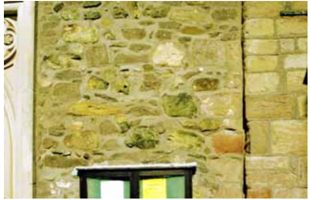
Figure 4. Mixed rubble stone. West front, St Laurence Church Stretton.
