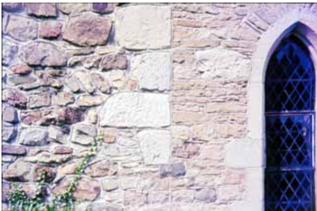
Figure 7. Predominantly Hoar Edge Grit. Norman nave left, 13 th Century Chancel right; Cardington Church.
