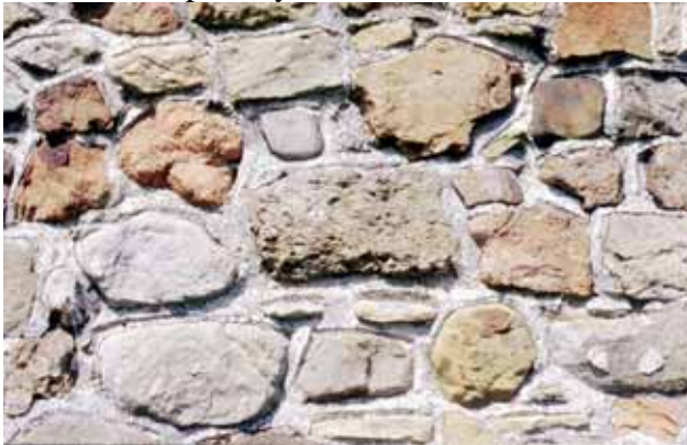
Figure 6. Geological mixture in Norman wall, Cardington Church.
