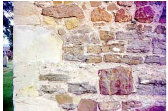
Figure 8. Rushbury Church, revealing Soudley Sandstone, Wenlock Limestone and possibly Hoar Edge Grit.
