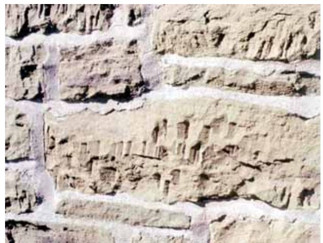
Figure 9. Rushbury Church, revealing Soudley Sandstone with 19 th Century tool marks - 'rustication'.
