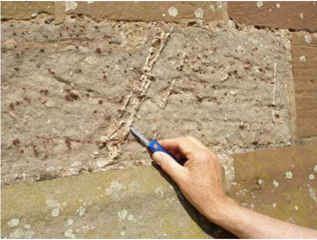
Figure 13. Block of buff sandstone of Upper Carboniferous age, reminiscent of the Big Flint Rock, in the wall of St Michael's Church, Lilleshall, containing prominent elongated white crystals of barytes.
