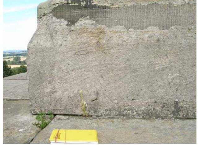
Figure 15. Block of Upper Carboniferous (Middle Coal Measures) sandstone, part of the plinth for the Duke of Sutherland's Monument, Lilleshall.
