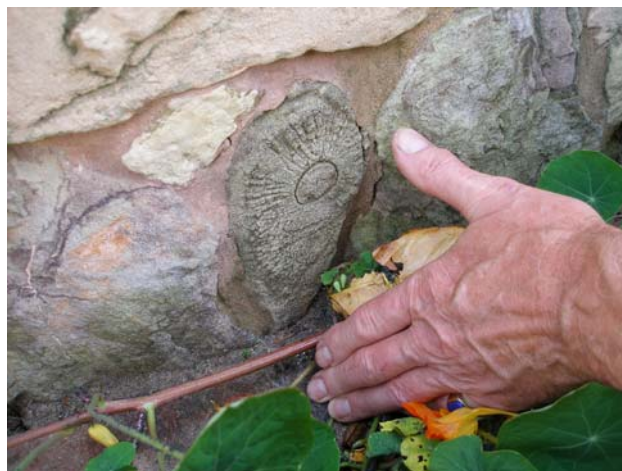
Figure 18. Large rosette of barytes employed as an ornamental feature in a garden wall, Lilleshall.
