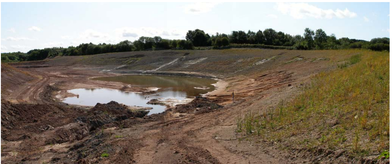
Figure 6. The now disused part of the workings between Hadley Road and the main railway line [SJ 680 116]. The on-going influence of groundwater can be appreciated with seeps flowing into the site beneath the cover of superficial glacial sediments, causing spring sapping and gully erosion. Water inflow is also occurring from deep within the Coal Measures, rising through fissures and old mine workings into the deeper levels of the site.
