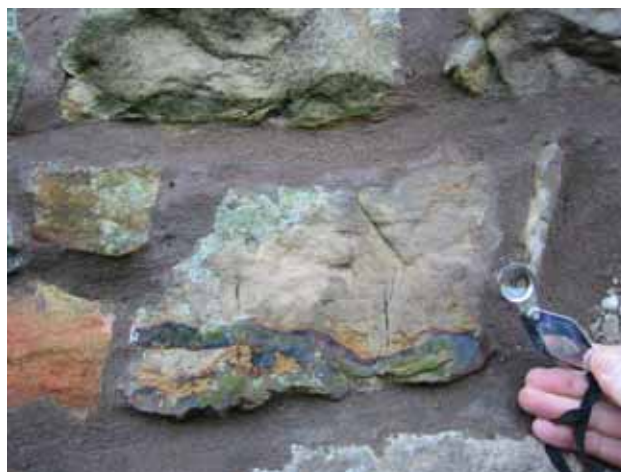
Figure 5b. Building stones at Upper Woodrow Farm – Coal Measures sandstone with ironstone (bands of grey siderite).
