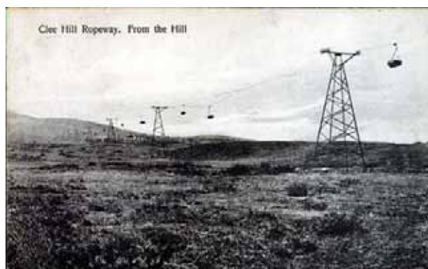
Figure 39. Aerial ropeway for transport of dolerite from Magpie Quarry (Field & Mackay (1911)).
