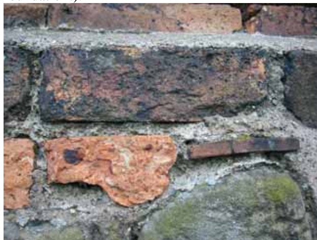
Figure 14. Bricks typical of those manufactured by the Knowbury Brick & Tile Works, with fragments of coal on their surface with which they had been dusted to facilitate removal from their moulds; Cleve Hill village.
