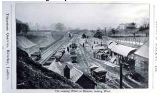
Figure 26. Bitterley Wharf exchange sidings just west of Locality 22, where quarried stone brought down by the incline railways was transferred to trains destined for the main line railway (Field & Mackay (1911)).
