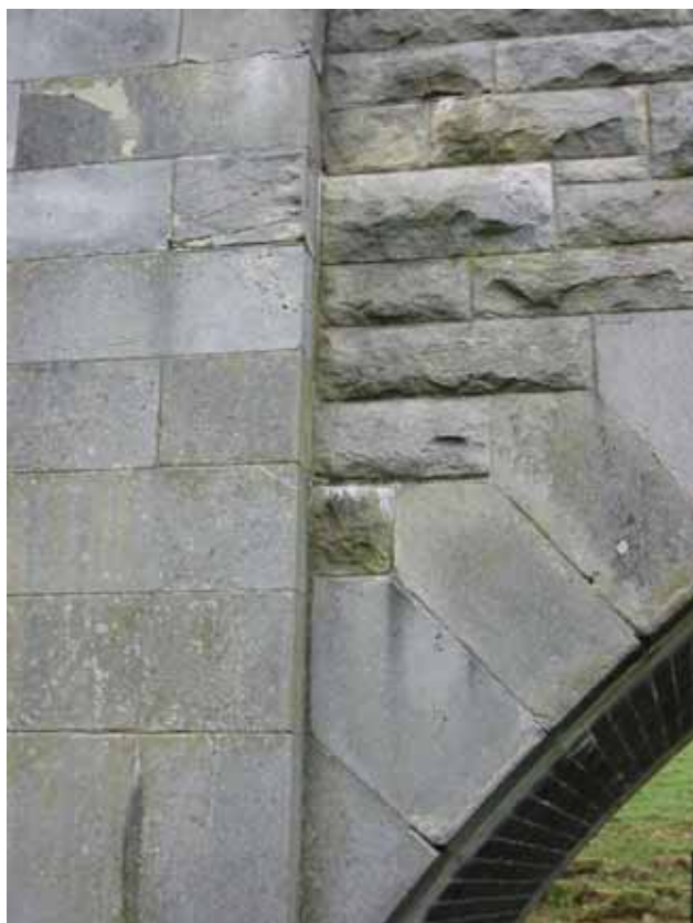
Figure 6. Sandstone ashlar in Elan Aqueduct.
