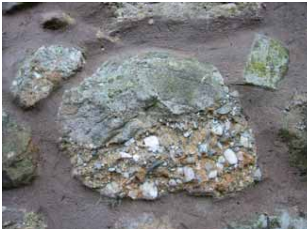
Figure 5a. Building stones at Upper Woodrow Farm – Cornbrook Sandstone.
